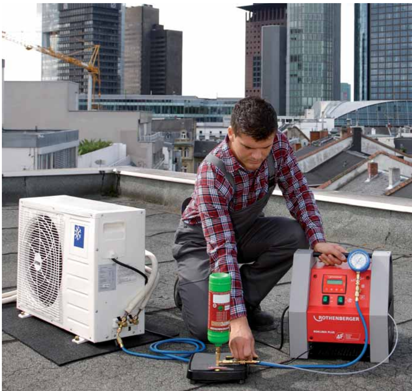
ROKLIMA PLUS 4F in use (evacuation and charging)
