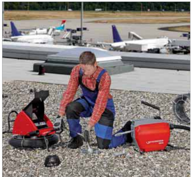
Inspection of a rain downpipe gutter
