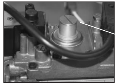
Governor adjustment screw under cover cap (SIT Nova 822)
