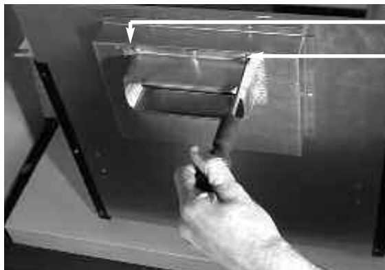
4 off Flue Spigot Fixing screws
